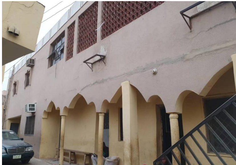
Figure 7: Showing the arrangement of windows and solar shading red bricks in the green building in Gwale LGA, Kano (Field Survey, 2020).
