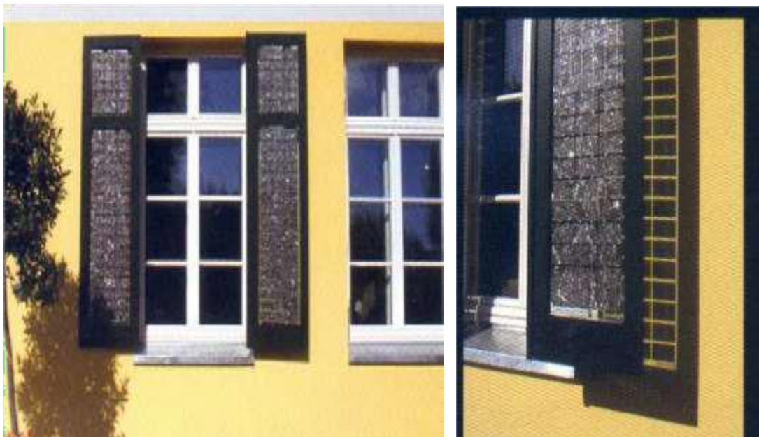
Figure 4.33: Use of PV in solar shutters, Germany (Gemicioğlu, 2011)
