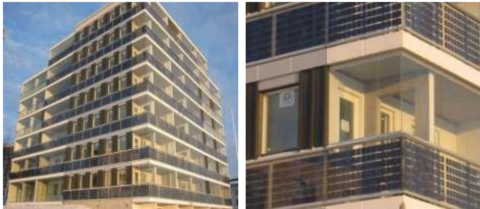
Figure 4.35: Using PV's in building railings, Finland (Gemicioğlu, 2011)
