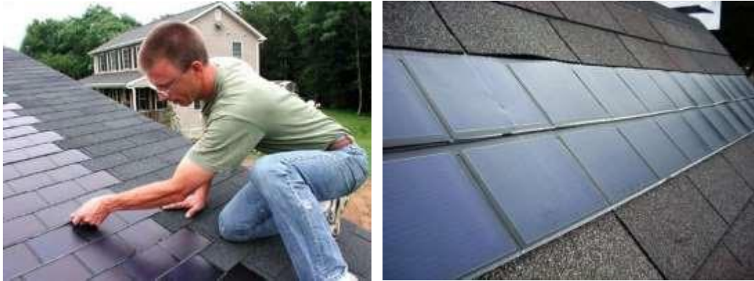
Figure 4.12: Shingle PV on the roof (Gemicioğlu, 2011)
