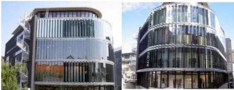
Figure 4.29: Vertical sun breaker curtain wall example (Yücel, 2016)
