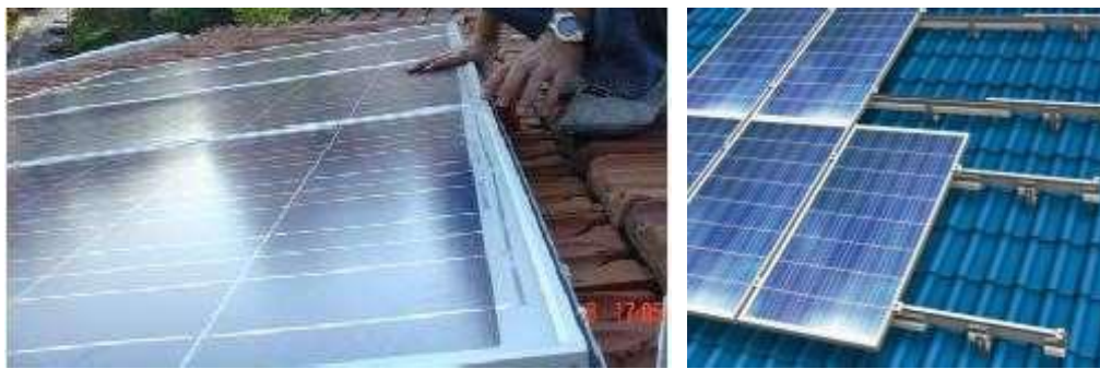
Figure 4.10: Using PV with an additional structure on the roof cover (Gemicioğlu, 2011)
