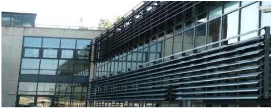
Figure 4.28: Horizontal solar shading (Yücel, 2016)
