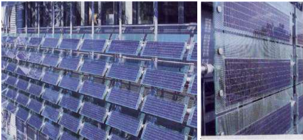
Figure 4.31: Using PV as a moving shading element (Gemicioğlu, 2011)
