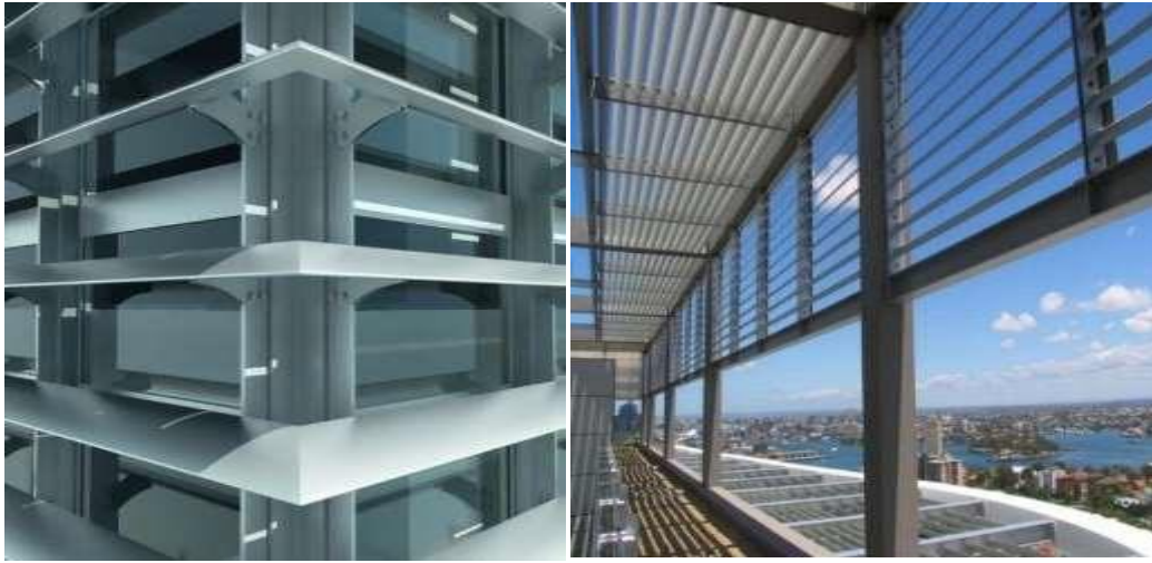
Figure 4.30: Fixed sunbreak facades (Yücel, 2016)
