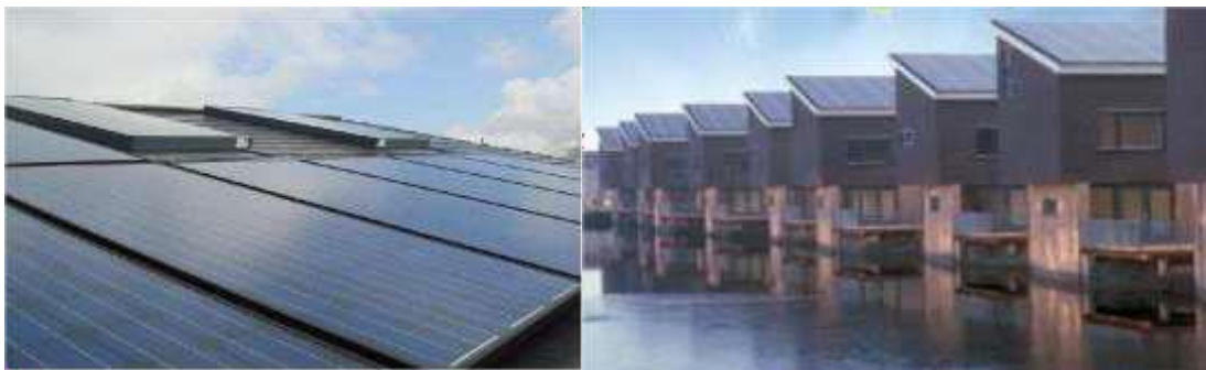
Figure 4.11: Use of PV integrated with roof cover (Gemicioğlu, 2011)
