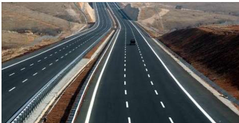
Figure 2.1: A highway example in Iraq (Erbil-Makhmour Highway) (Anadolu Agency, 2018)
