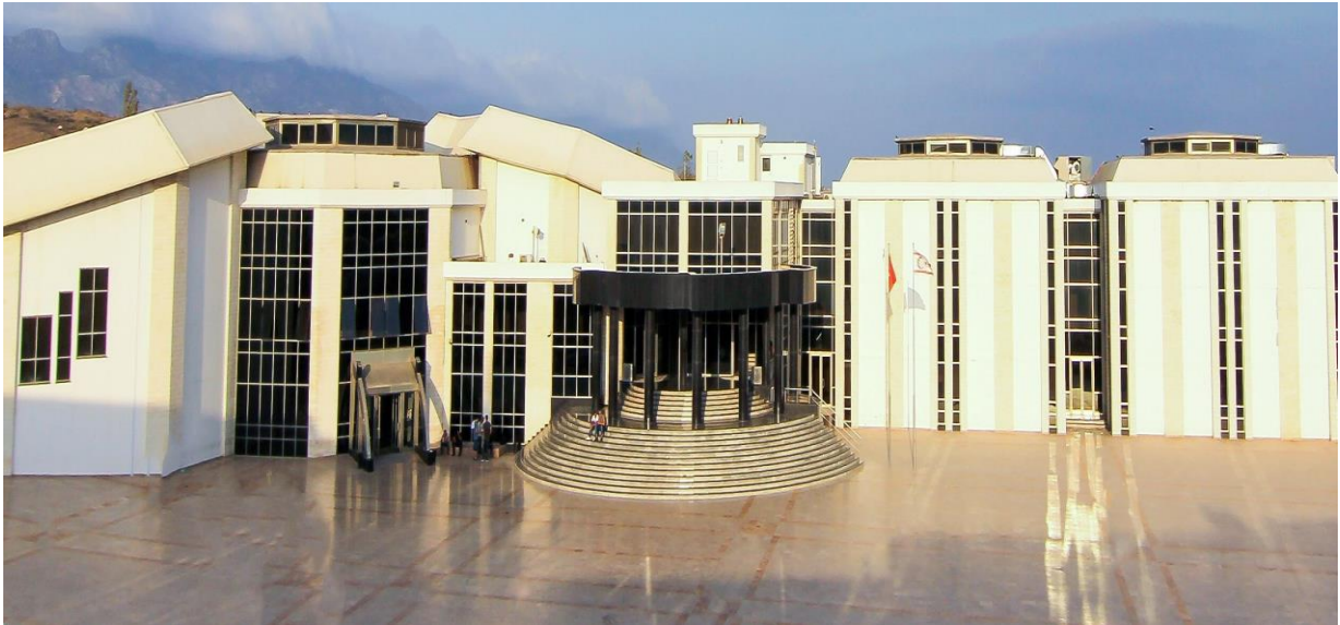
Figure 3. 11: Near East University Grand Library front view (Photo: L, Arafa, 2021)
