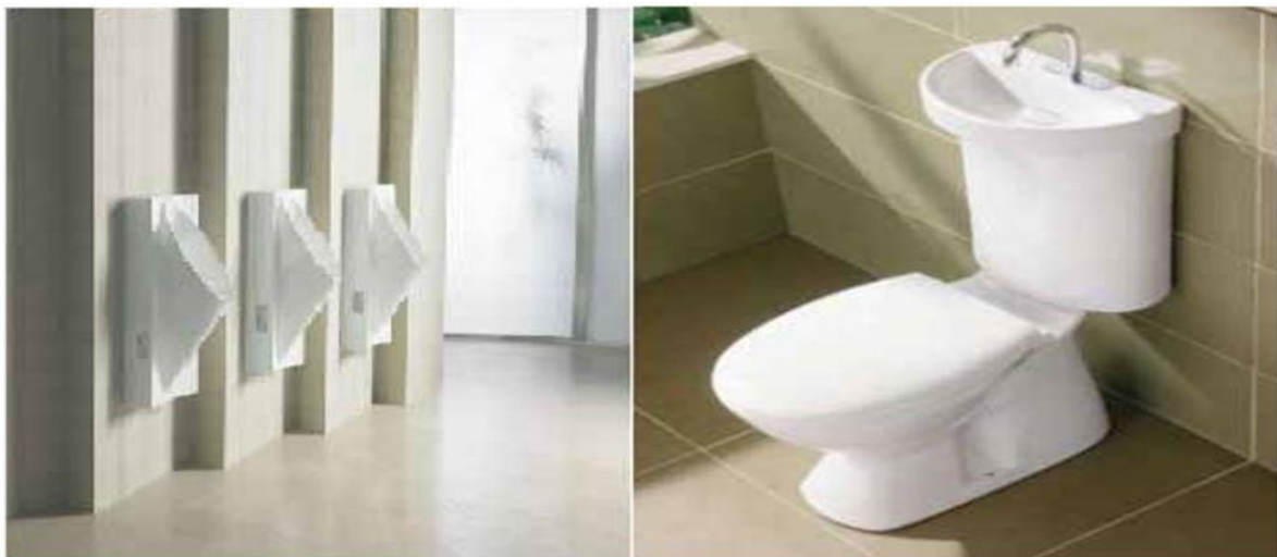
Figure 3. 8: Sustainable restroom fittings in the AMQF building (Photo: L, Arafa, 2021)
