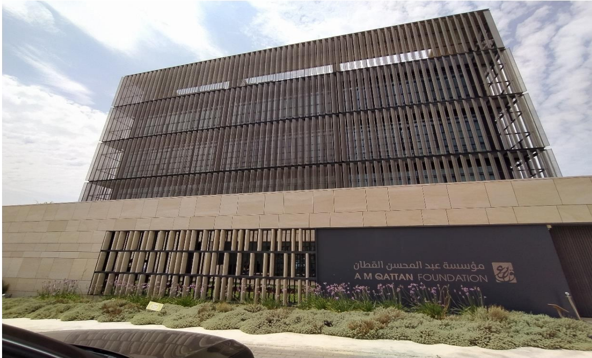
Figure 3. 1: Front view of the AMQF building (Photo: L, Arafa, 2021)
