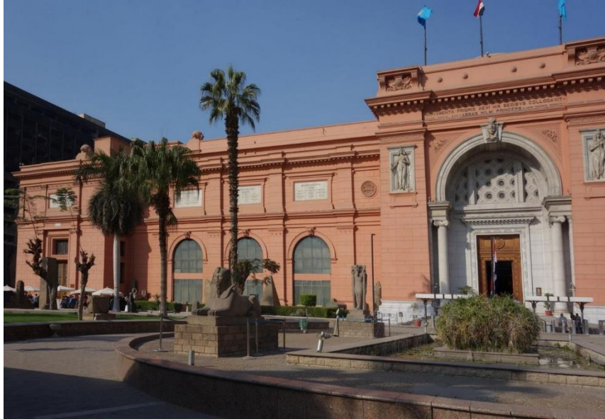
Figure 4.1: Egyptian Museum façade today (Asfour, 2014).
