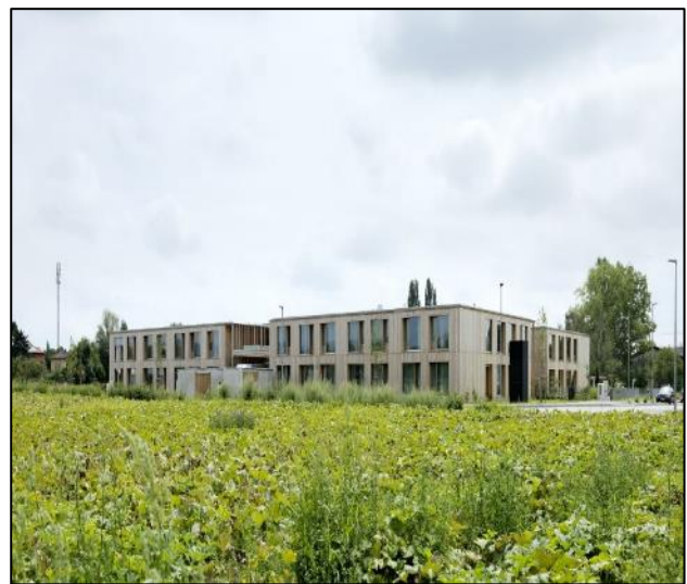
Figure 1.6: Area view of nursing home (arcdaily.com,2014)
