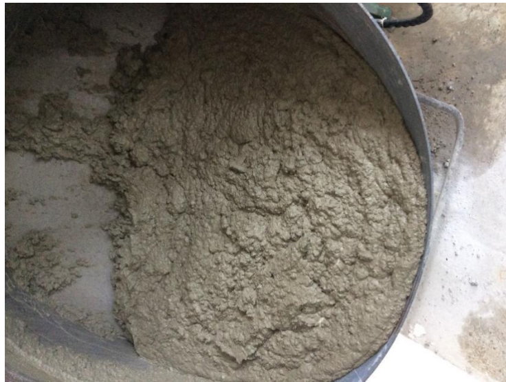
Figure 3.11: The concrete mixture
