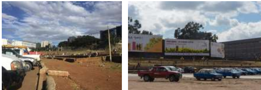
Figure 5. 7: Parking areas in Addis Ababa (February 29, 2020)
