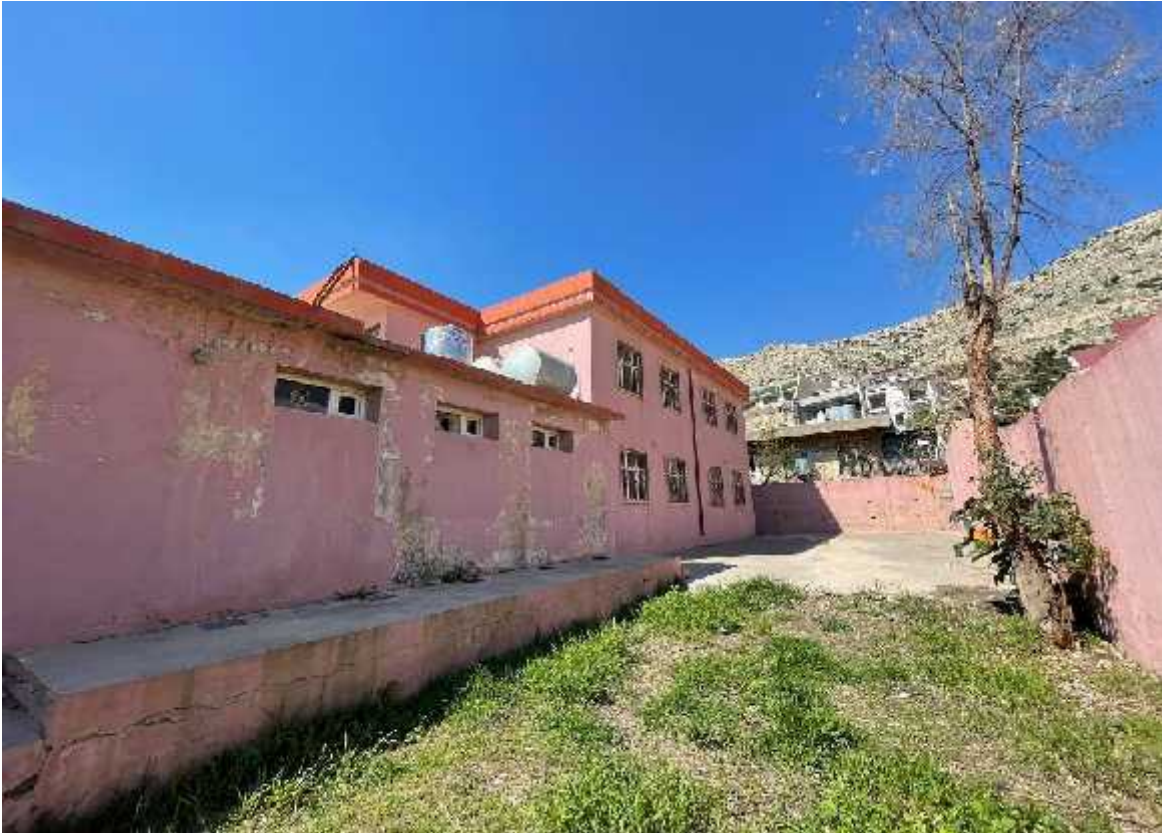
Figure 4.8: Showing the only unpaved area with dried tree and scattered grass
