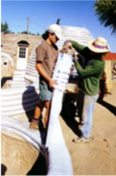
Figure 2.15: USA, California, cal-earth – filling superadobe (Khalili, 2012)
