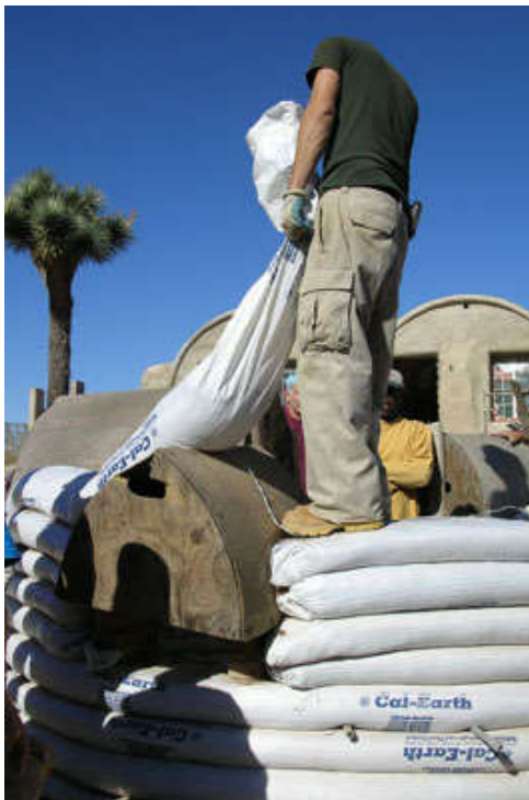
Figure 2.16: USA, California, cal-earth – tamping the tubes (Khalili, 2012)
