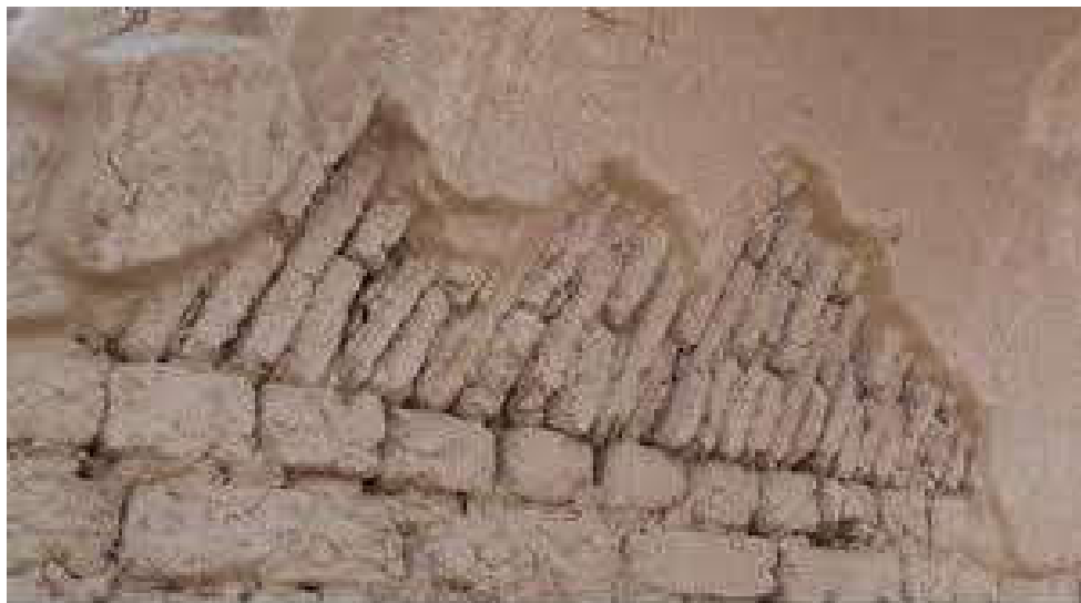
Figure 2.23: Mud-bricks laid tilted in Egypt (Beck,1987)
