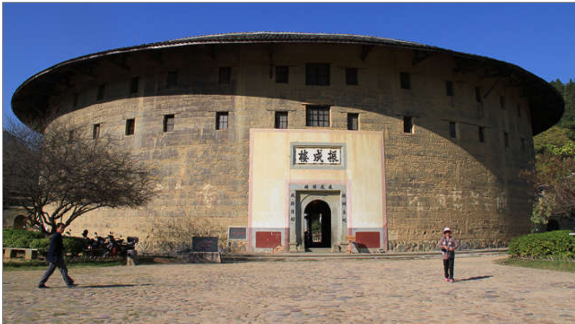
Figure 2.8: China Fujian province – village/house of Hakkas clan (Leslie, 2019)
