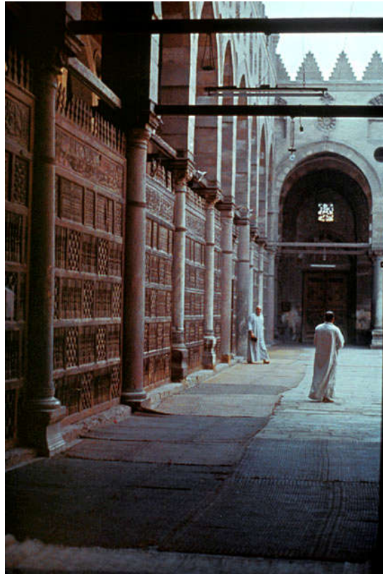
Figure 3.6: Wooden mashrabiya in masjid Altinbugha al-Maridani, Egypt (Williams, 1978)
