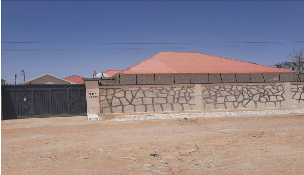
Figure 23: Typical house for the family in Banadir region areas
