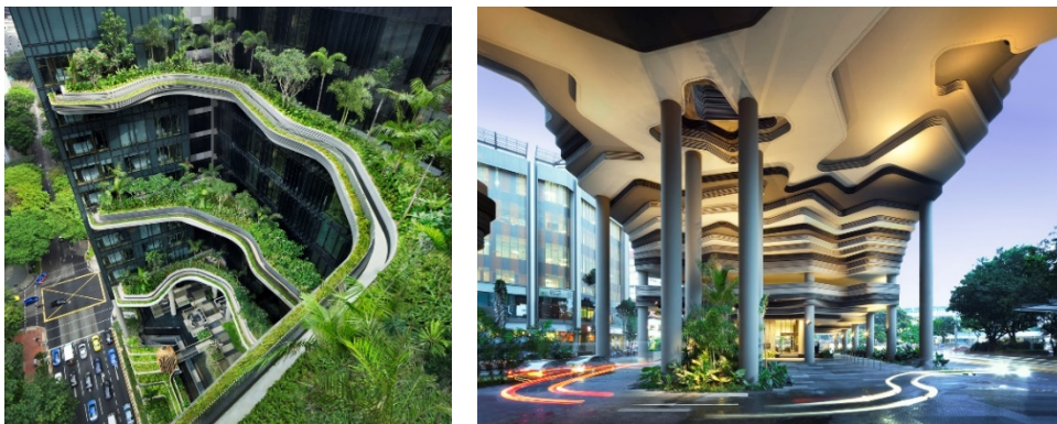
Figure 2: PARKROYAL on Pickering. (Bingham, 2013)
