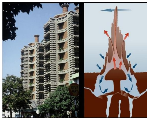
Figure 10: Eastgate building, Zimbabwe, Simulation of termite's mounds (Shahada et al., 2014).
