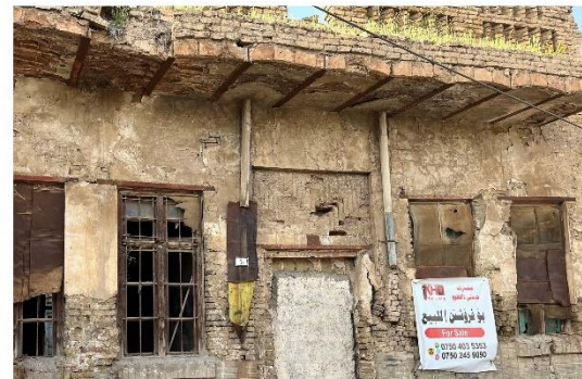
Jack arched slab and cantilever
