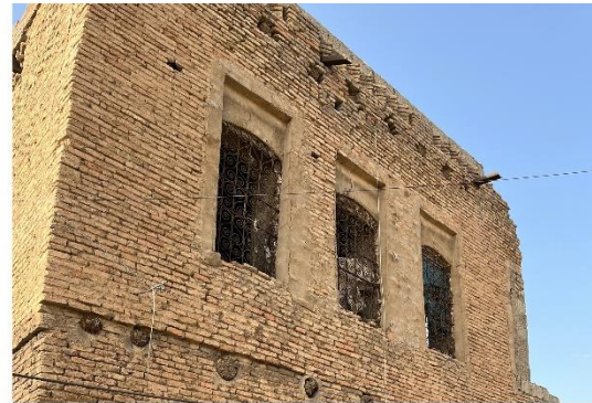
Arched window opening &amp; iron fenced window
