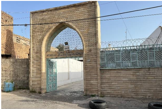
Arched door opening
