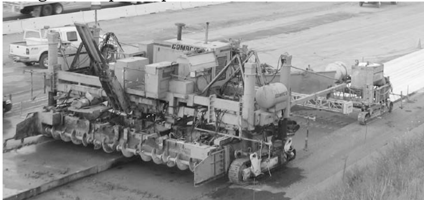
Figure 3.35: Large Grade Trimmer/Reclaimer/Paver
