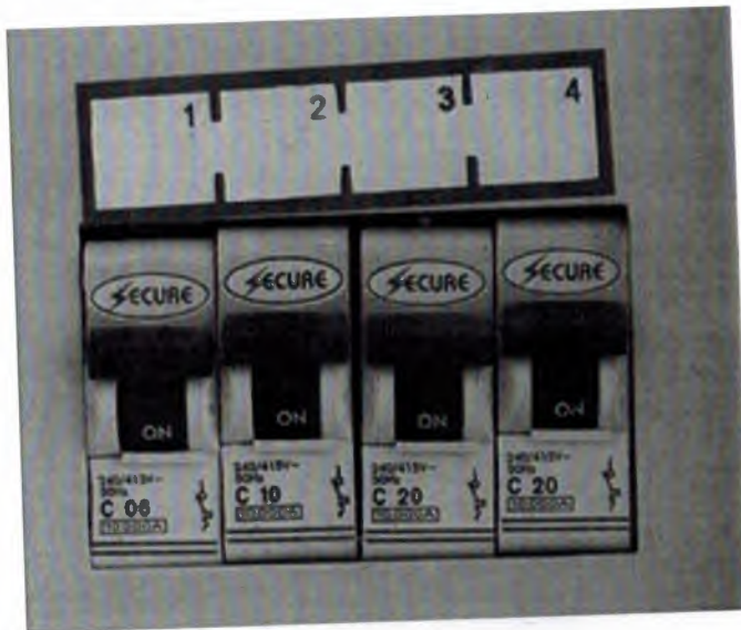
Fig.8: Miniature Circuit Breaker
