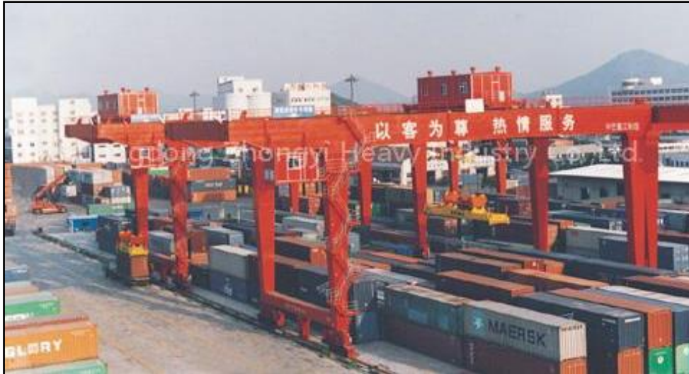
Figure 4.18: Rail-Mounted Yard Gantry Crane
