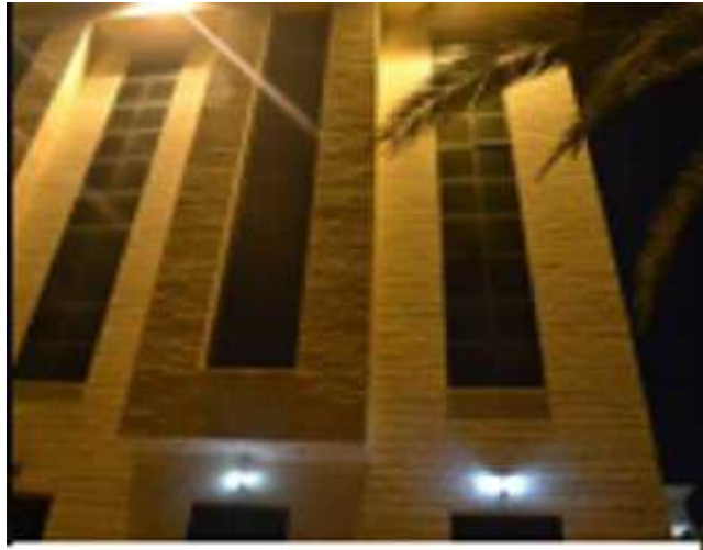
Figure 4.20: The Building of the Palestinian Retirement Authority, finishing material (James, 2013).
