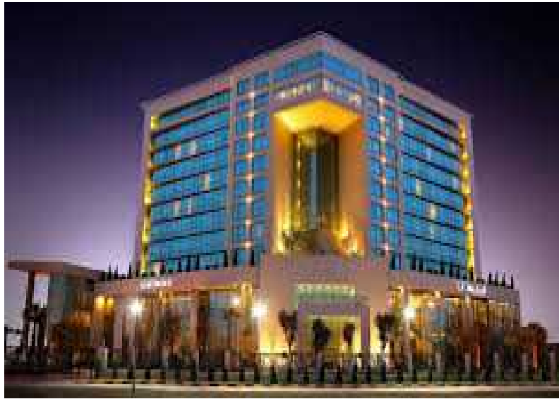
Figure 4.31: Rotana Hotel, Erbil, finishing material.
