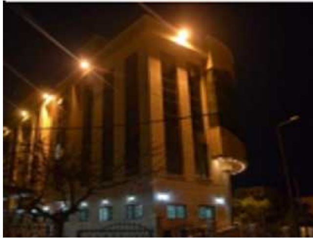
Figure 4.18: The Building of the Palestinian Retirement Authority, colour (Baker, 2015)
