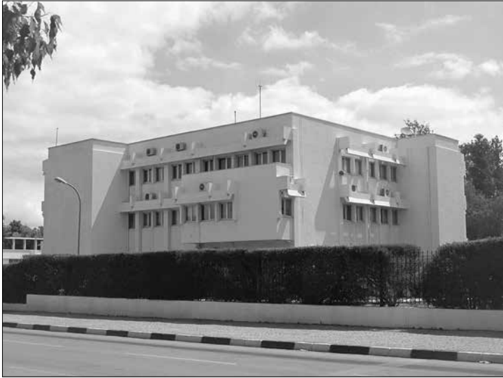
Figure 2 The Turkish Embassy Building, 2010.
