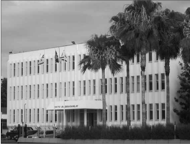
Figure 3 Prime Ministry Building, 2010.
